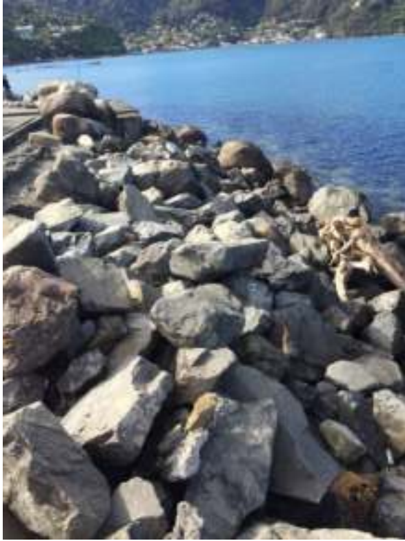
Photo 2. Riprap rock revetment little blue penguin habitat within the project site.
